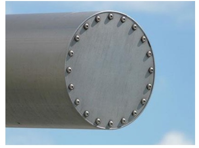
Rivets on end of a metal pipe
